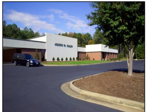
STAPLES MILL 8510 Staples Mill Road Richmond, VA 23228
