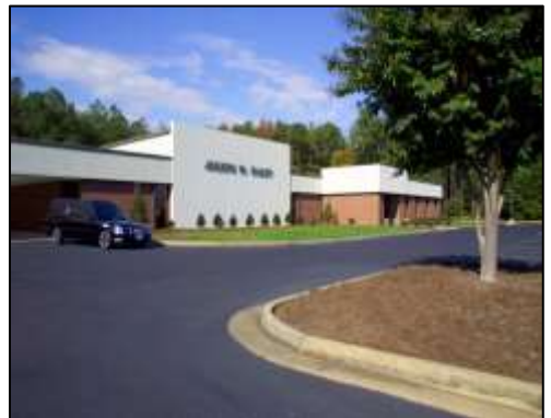
STAPLES MILL 8510 Staples Mill Road Richmond, VA 23228
